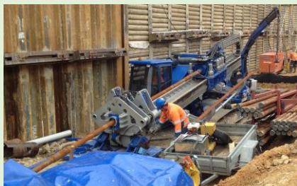
Interlocking rods being screwed through from the trench to Cambridge Tce for the pilot hole
