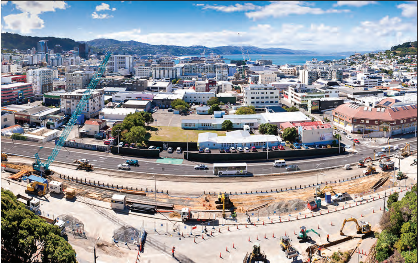
April 2013: This panoramic photo shows earthworks for the new tunnel and road to go underneath the National War Memorial Park and also shows where the road in Buckle Street was diverted in January 2013 to run beside Mount Cook School.
