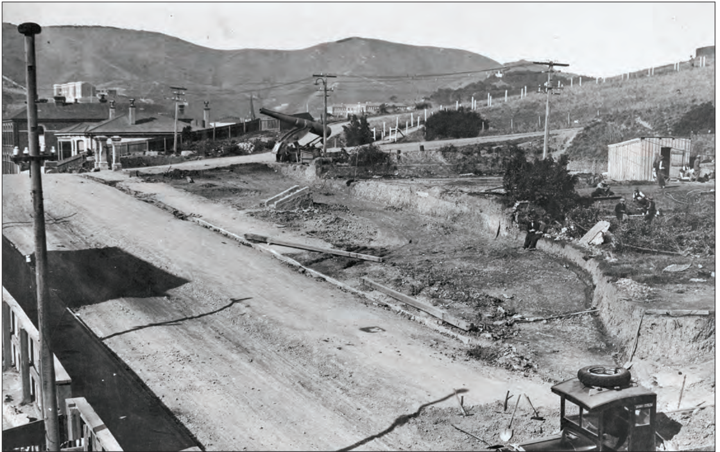
May 1930: Roadworks on Buckle Street with a cannon visible at the barracks gates. Source: Alexander Turnbull Library; Ref: 1/2-075035-F. Photo: Evening Post newspaper.
