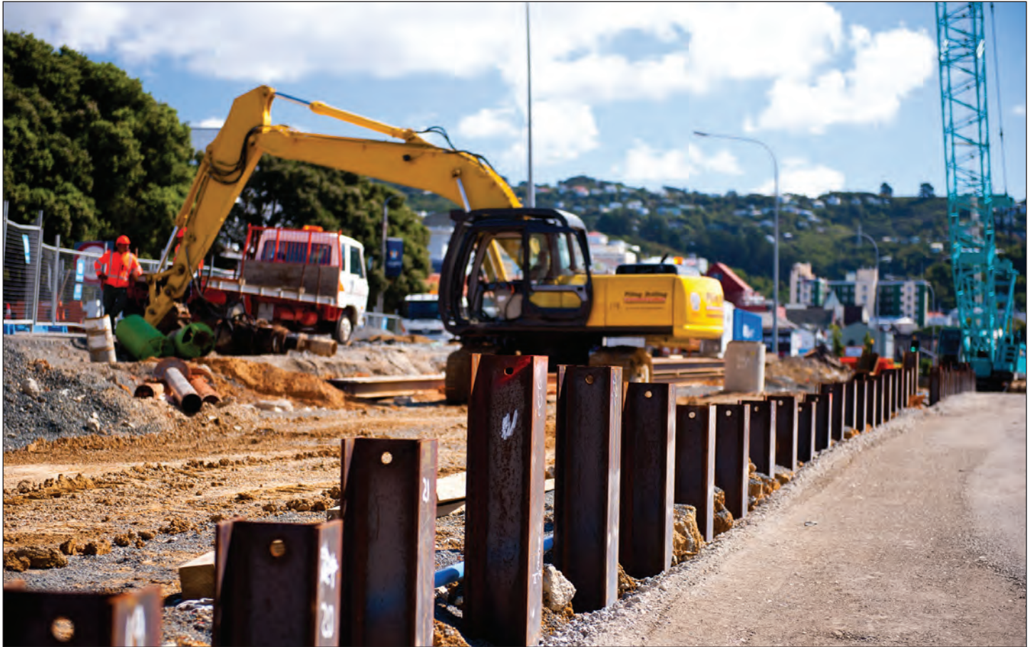
2013: King posts are driven into the ground to be the supports for retaining walls when the trench is dug for the National War Memorial Park Underpass.
