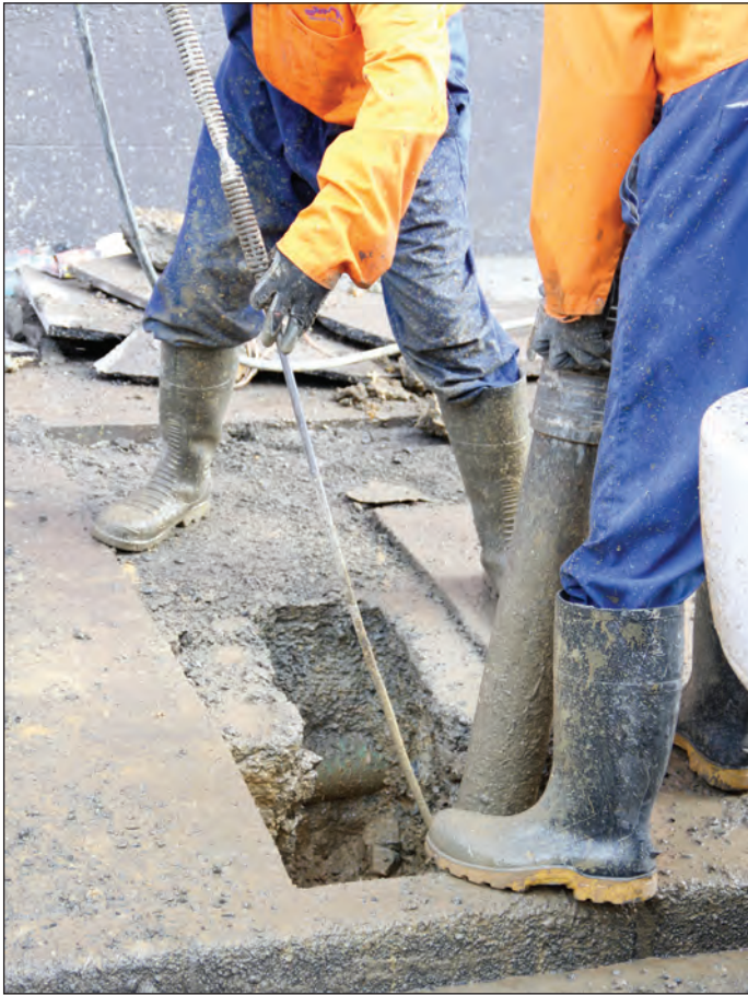
2013: A careful operation is needed to move the pipes out of the way. At left, the vacuum cleaner sucks up slushy soil with a hose. At right, the ground at the sides is held in place by retaining walls so workers can put in a new water pipe.
