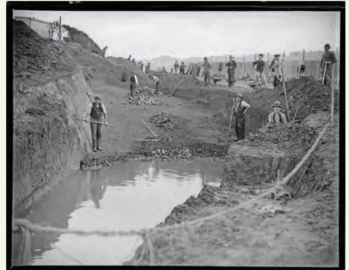
1931: Labourers carry out earthworks near the site for the National War Memorial Carillon and Dominion Museum. Source: Alexander Turnbull Library; Ref: 1/2-090207-G; Photo: Evening Post
