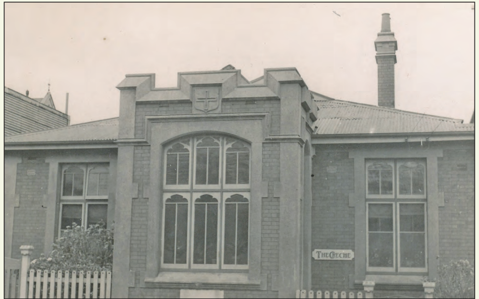
Front view of the former Home of Compassion Crèche.
