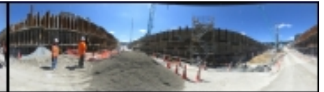
In and around the trench (2 images) [4]
