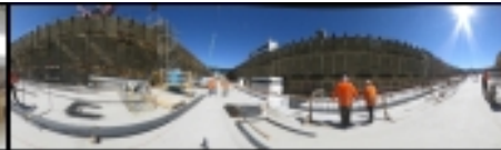
In the trench (2 images) [3]
